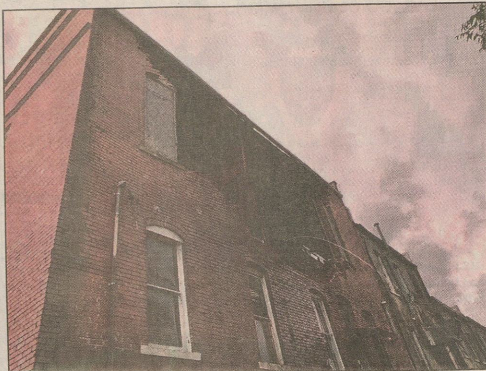
The tornado blew the back of the brick building out, leaving a hole in the office of Nicholas Phillips on the top floor.
